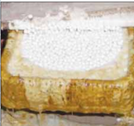
Figure 1: Long-time high temperature results in serious carbonisation.
