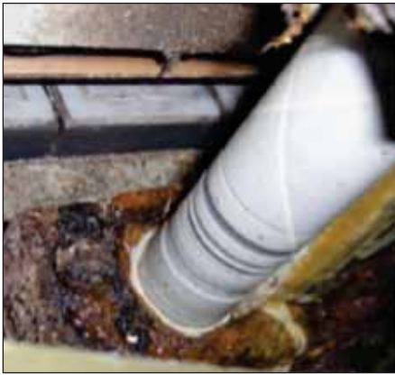
Figure 3: Carbonised particles block up the glue quantity adjusting system.
