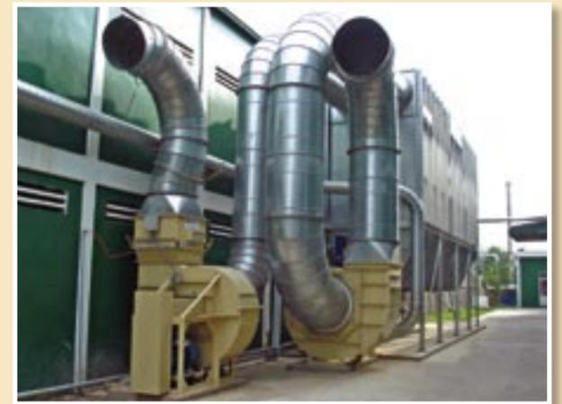
High efficiency fans and Moldow MHL filter system
