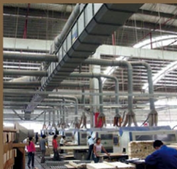
Moldow's Transflow system allows maximum flexibility to change the production layout.
